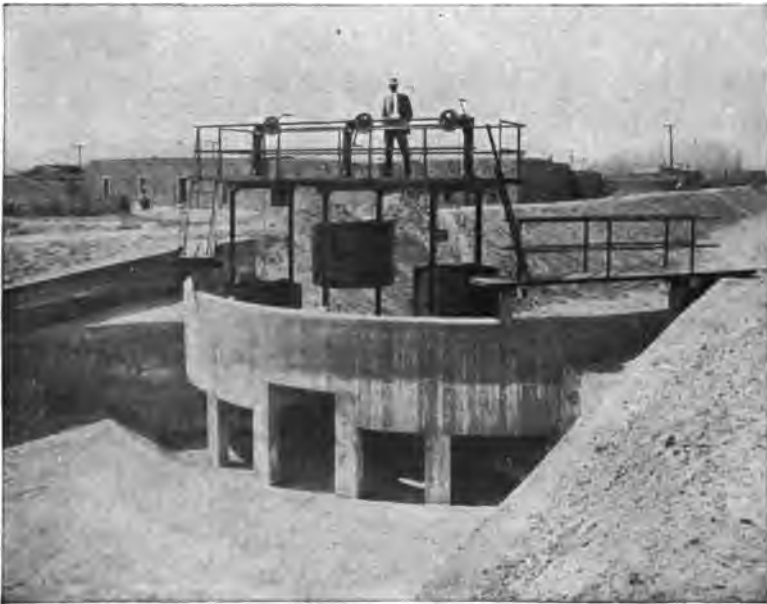
FIG. 126.—Cylinder Drop on Franklin Canal, Rio Grande Valley, Texas.
